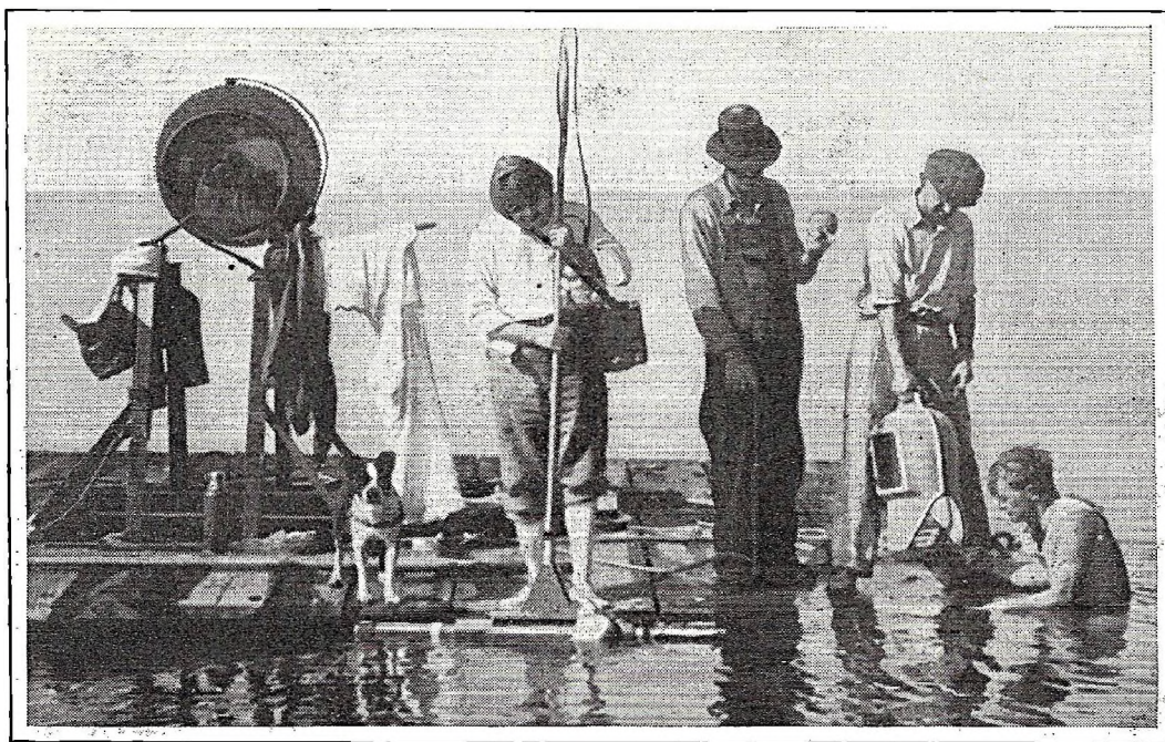
Raft equipped with radio divining rod apparatus and air pumps, is used on Lake Ontario to locate old cannon and other relics of early warfare, to be used in re-equipping Fort Niagara. Pump man is holding cannon ball brought up by diver.
